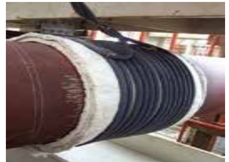
Post Fabrication Stress Relieving
